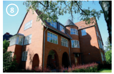
8 International House. Erected 1911-1912, designed by Heinrich Straumer as an entomological museum. Since 1953, used by Freie Universität. Since 2015, part of the International Affairs Division: home to liaison offices of international partner universities.
