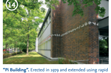
14 "Pi Building". Erected in 1979 and extended using rapid construction methods. In 1980, the Institute of Mathematics moved in.
