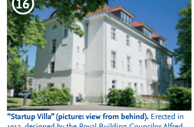
16 "Startup Villa" (picture: view from behind). Erected in 1912, designed by the Royal Building Councilor Alfred Koerner as the Astronomical Computing Institute. 1973-1994 home to Executive Board of Freie Universität. Since 2015, headquarters of Freie Universität's start-up program, Profund Innovation.
