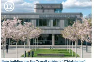
12 New building for the "small subjects" ("Holzlaube", wood cabin). Extension of the Rost- & Silberlaube, erected in 2015, designed by Florian Nagler. Home to 14 "small subjects" and a "campus library" that integrates 24 institute libraries.
